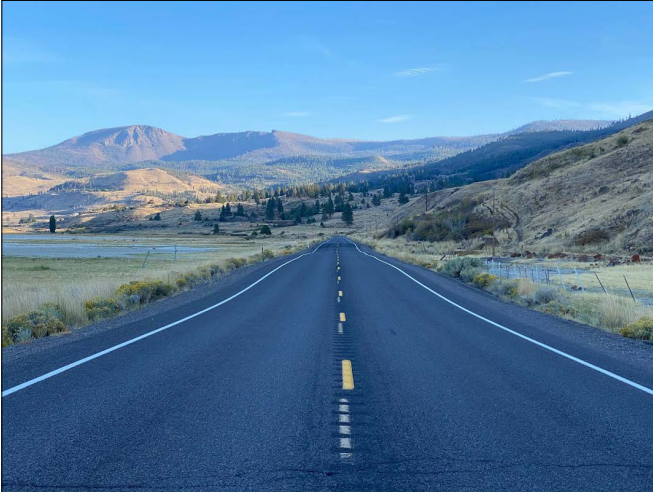
Figure 8. Road in Lake County, OR.
